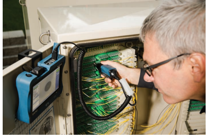
Figure 6. Fiber inspection: All connections must be clean and free of contaminants
